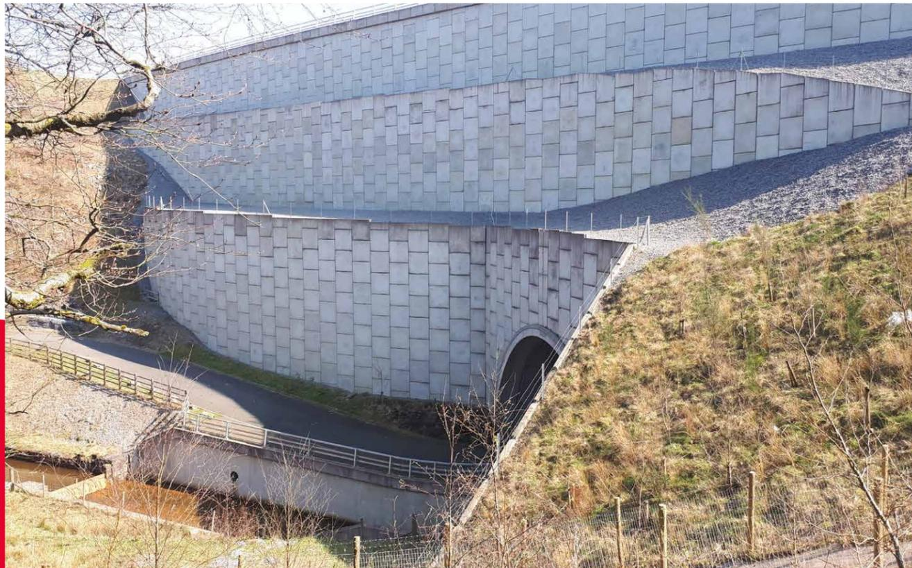
Reinforced Earth technology provides an amazingly efficient solution for very high retaining structures. The precast concrete facing panels used have a maximum thickness of 160mm. This offers huge environmental benefit from lower carbon emissions when compared to other solutions such as cast in place reinforced concrete walls. It also reduces the transportation to site by almost 90% providing environmental safety and community benefits.
