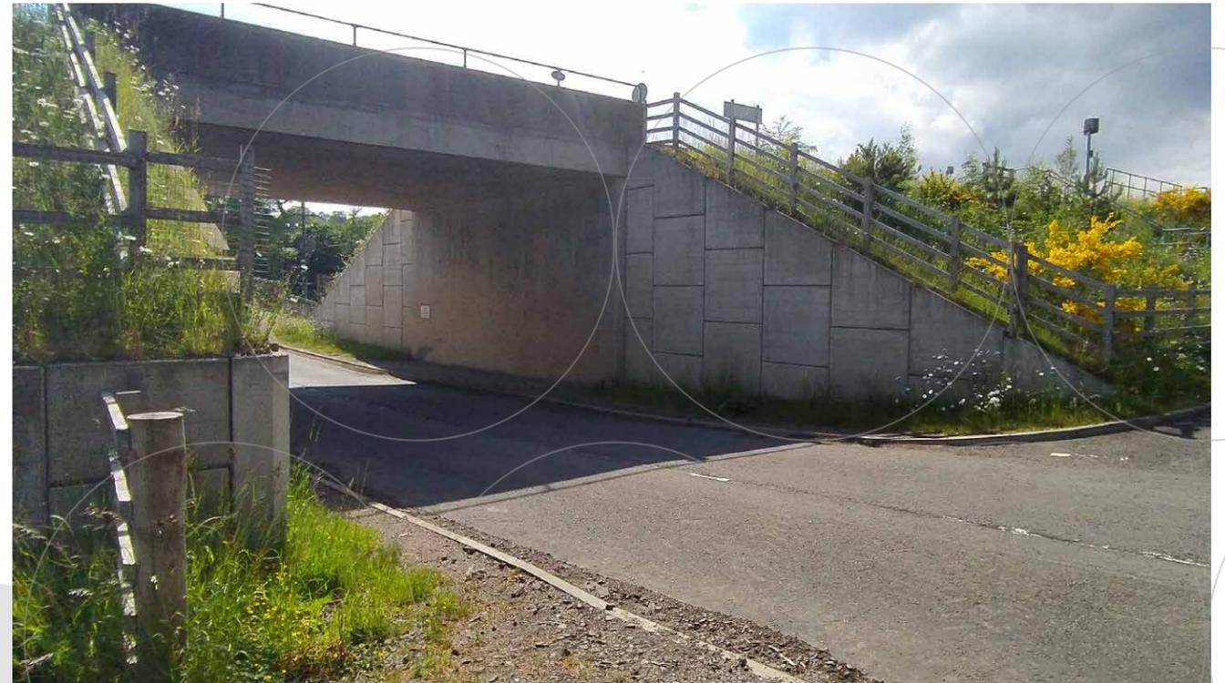
GeoStrap® is ideal for use in road applications as the fill used around the strips has no limitation to its salt content.
